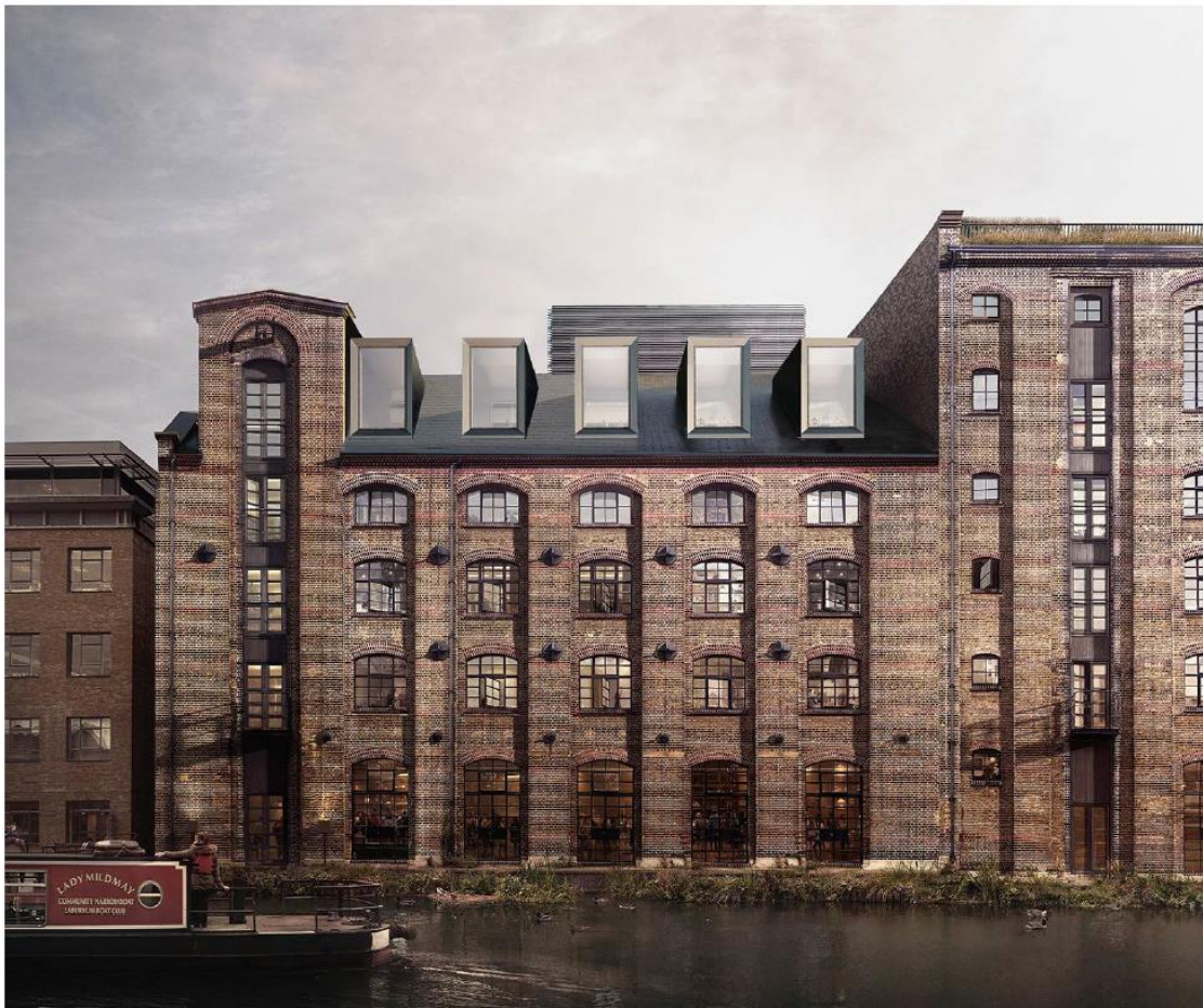
Building B (No. 10 Regent's Wharf) – canal-side elevation
